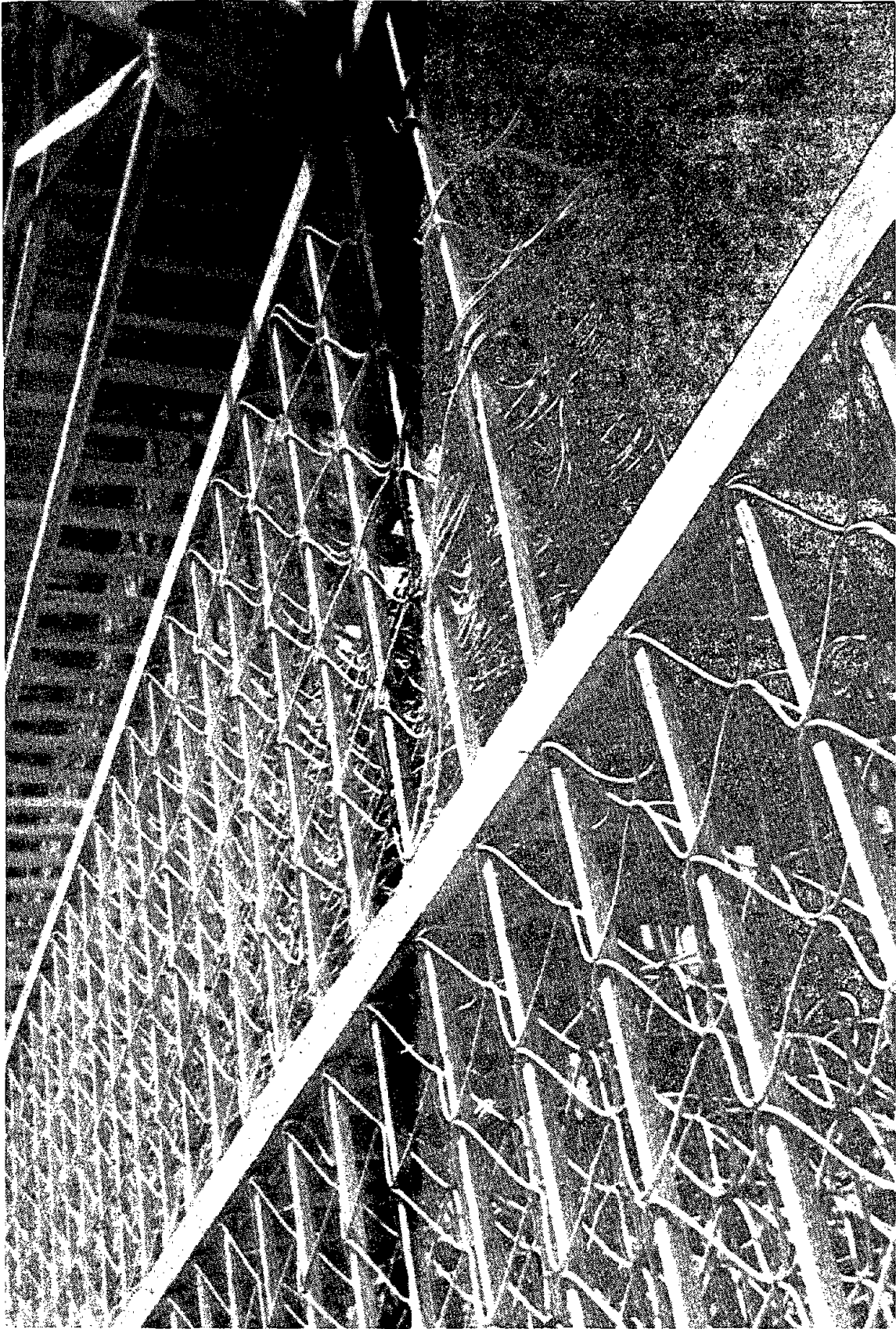
Figure 5. Three-Dimensional Detonating Cord Weave Installation (Typical)
